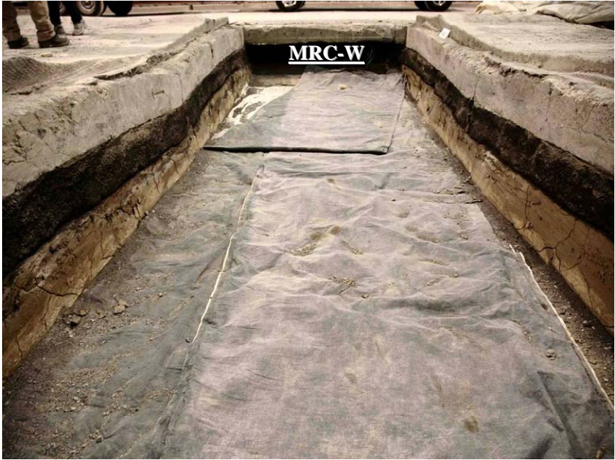
MRC Trench – West End
